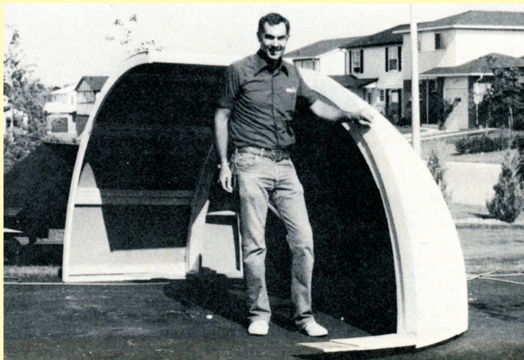
The author, Jack Newton, stands beside the partially completed dome of his new observatory.
