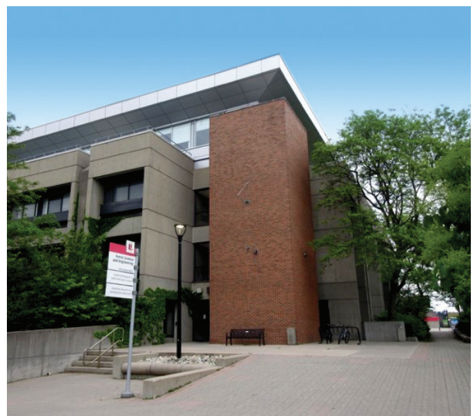
Figure 2 — R.M. Petrie Science and Engineering Building, York University, Toronto (Photo by DCM)
