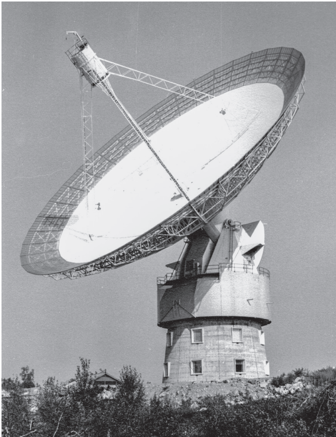
Figure 12 — The 46-m ARO telescope and at left the control building, at ARO in 1968. Receivers are available at three wavelengths, offering increasingly sharp pencil beams: 9-cm (9'), 4.5-cm (4.2'), and 2.8-cm (2.7'). When commissioned, this is the third-largest fully steerable telescope in the world, after Jodrell Bank and Parkes. Receivers may be mounted at both the prime focus and Gregorian focus.
