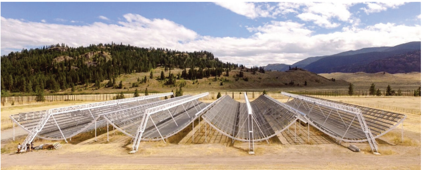
Figure 1 — The CHIME Telescope is designed to provide a large collecting area while also surveying a large part of the sky above the telescope, allowing efficient surveying of the radio sky for FRBs. Image Credit: CHIME
