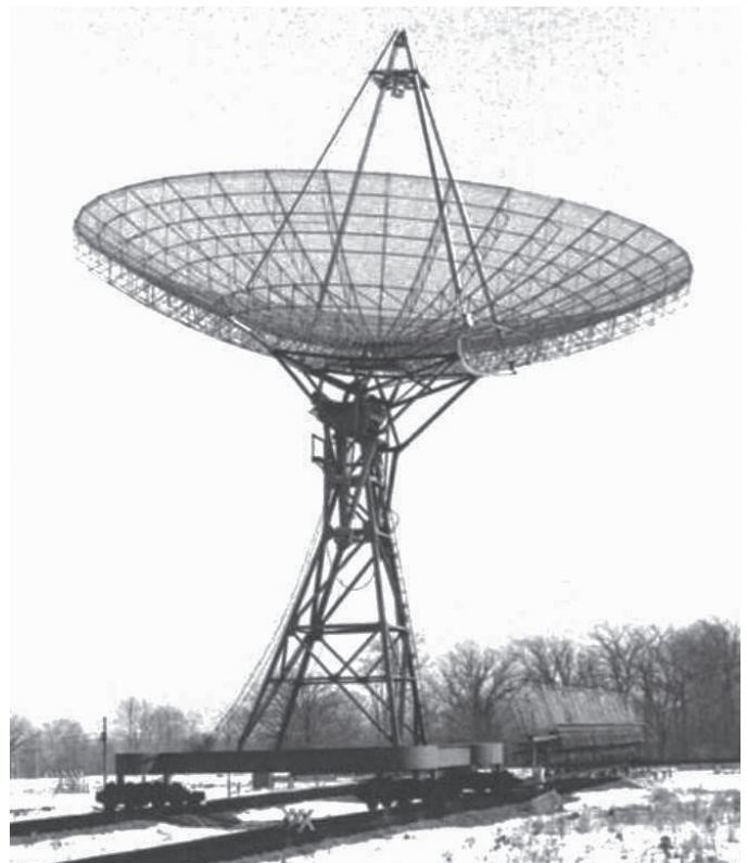
Figure 10 — The QRO 18-m dish on E-W rails in 1969. Plans for a second dish to form an interferometer were never implemented. In the background to the East sit the twin arrays for 35-cm wavelength built by the Electrical Engineering Department.
