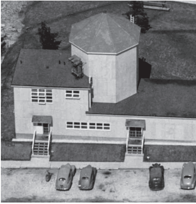
Figure 5 — Celestial Navigation Trainer Building at Lakehurst, New Jersey, Naval Air Station, July 1945. Image: National Archives photo, 80-G325735. Sourced from Smithsonian National Air and Space Museum (accessed 2020 March 20) https://airandspace.si.edu/stories/editorial/women-guided-way-simulated-sky-during-wwii
