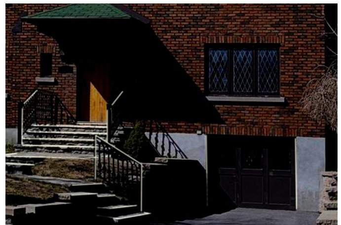
Figure 6 – Reflective paint to highlight hazards and features. Some hazards are identified by the irregular shadows they cast. However at night these shadows can be indistinct—even with flashlights. Highlighting these features with reflective pain (white or yellow) will make them more visible with less artificial light—even under moonlight. (Simulated image)
