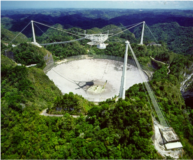
Figure 1 – (left) The Arecibo radio telescope seen before its collapse. The 305-m dish is nestled in a natural sinkhole in Puerto Rico. The secondary feed structure is supported over the dish by three cable towers. (right) Image of the secondary feed structure collapsing onto the dish, captured during the collapse of the telescope on 2020 December 1. Image Credits: Arecibo Observatory, a facility of the US National Science Foundation.
