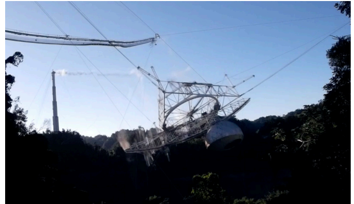
Figure 1 – (left) The Arecibo radio telescope seen before its collapse. The 305-m dish is nestled in a natural sinkhole in Puerto Rico. The secondary feed structure is supported over the dish by three cable towers. (right) Image of the secondary feed structure collapsing onto the dish, captured during the collapse of the telescope on 2020 December 1. Image Credits: Arecibo Observatory, a facility of the US National Science Foundation.
