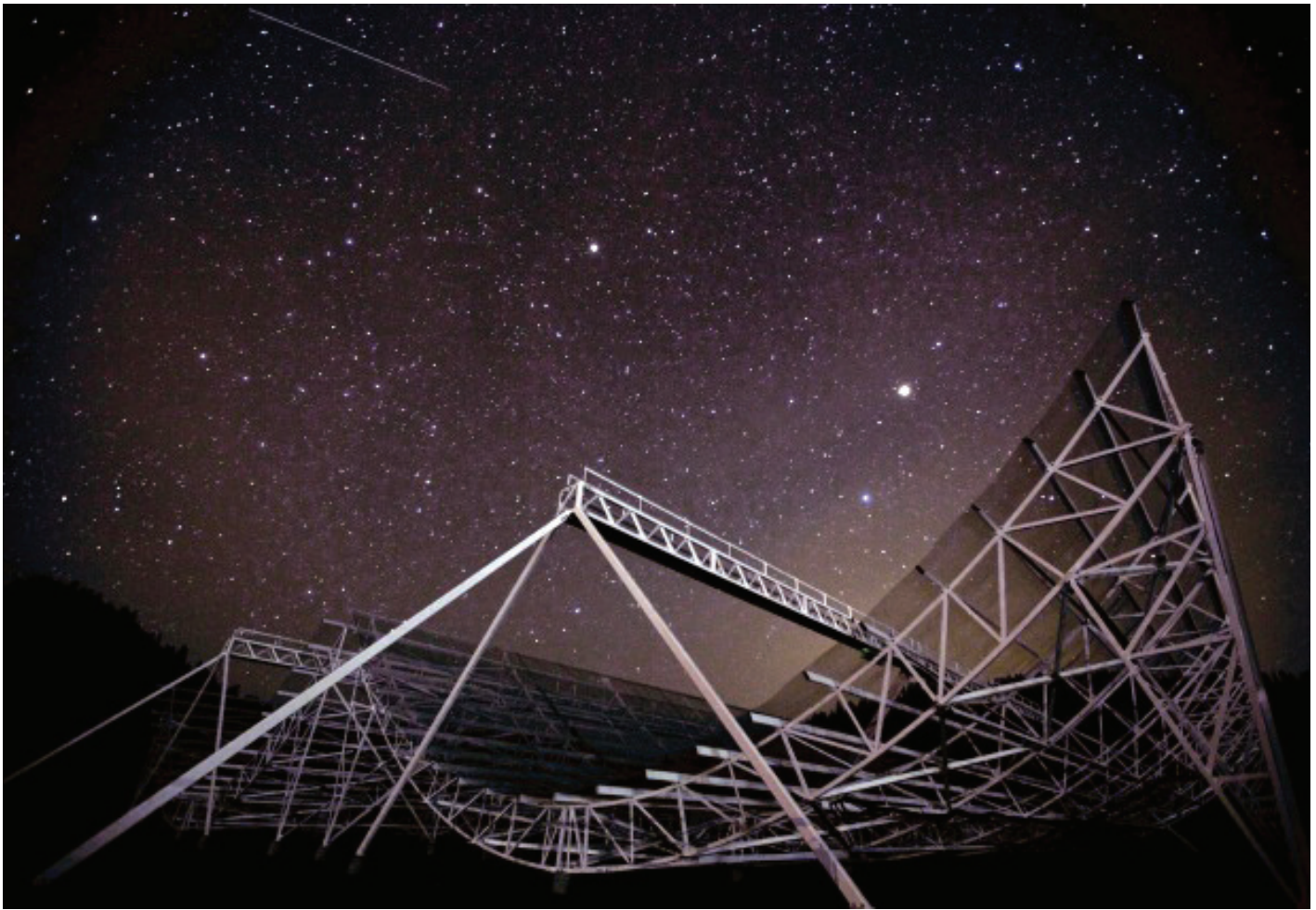
Figure 1 — CHIME: The Canadian Hydrogen Intensity Mapping Experiment is an innovative, cost-effective radio telescope, located near Penticton, BC. It has a collecting area the size of five NHL hockey rinks, but has no moving parts. The sky drifts by; powerful computers do the rest of the work. It was designed to map the neutral hydrogen in the early Universe across the northern sky, but it will also detect and study short-lived phenomena such as pulsars and fast radio bursts. Source: Dunlap Institute.
