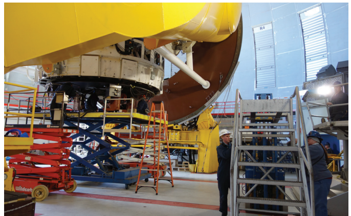
Figure 1 – CFHT staff begins the process of removing the primary mirror. The parallel red tracks are where the mirror cart slides under the primary.
