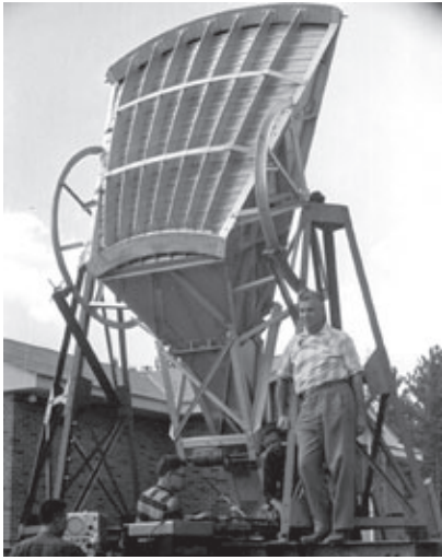
Figure 8 — An image showing preparatory work on the horn reflector antenna at the University of Toronto site of the Algonquin Radio Observatory. It was used to measure the absolute brightness of galactic emission at 707 MHz at the North Celestial Pole (reproduced courtesy of the Department of Astronomy & Astrophysics, University of Toronto).
