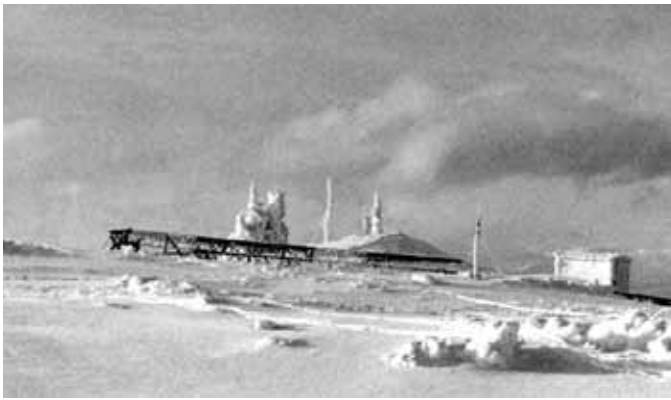
Figure 15 — The collapsed weather tower, 1968 January 16. Courtesy Library and Archives Canada. Pictorial record in RG48, Vol. 36, Folder 4.3.
