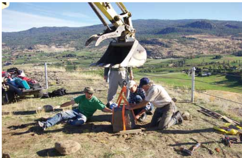
Figure 1 — A backhoe, assisted by (l-r) Jordy Bouillet, Jim Shaver, and Chris Purton, was used to align three holes drilled into the bottom of the ~225-kg heel stone with lengths of rebar that were cemented into the bedrock to firmly secure the markers.
