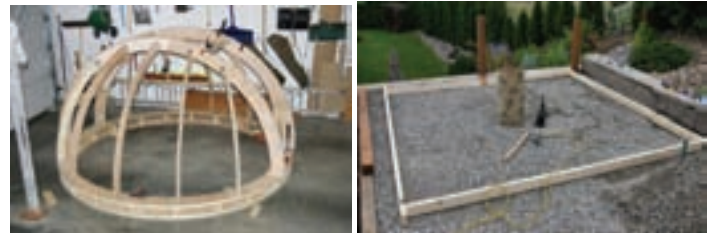
Figure 6 — Frame of the dome Figure 7 — Ground prepared for cement pad
