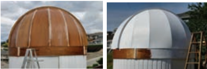
Figure 12 (left) — 1/4-inch mahogany plywood fastened and to be filled with Bondo and fiberglass Figure 13 (right) — Dome with several coats of ribs resin and paint.
