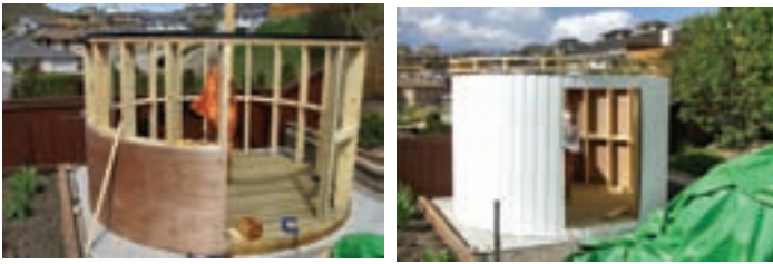
Figure 10 (left) — Applying 1/4-inch mahogany plywood Figure 11 (right) — Finished wall with vinyl siding and the dome base ring in place. Note the fence on the top of the wall, constructed at the insistence of my wife so that I would not fall again.
