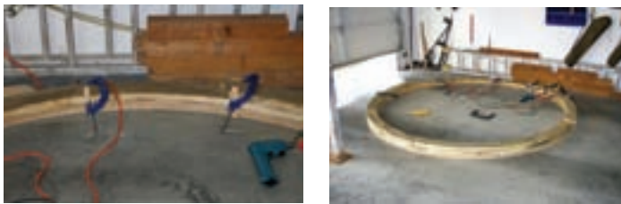
Figure 3 (left) — Fitting ring together Figure 4 (right) — Ring for base of observatory wall
