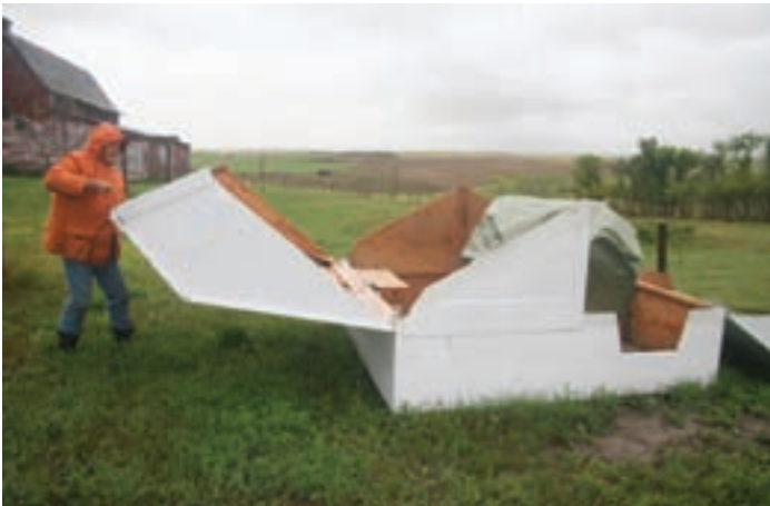
Figure 1 — Tenho Tuomi opens his clamshell observatory. The triangular end panels simply lift out and store in the open roof. The tarp is because it was raining.
