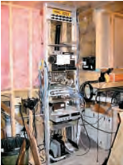
Figure 7 — “HAL 2003.” The rack contains the operational heart of Radio Jove, the meteor detection system, and video and network distribution for the building and all the piers.
