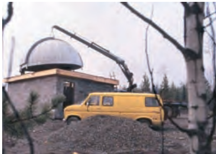
Figure 4 — The dome for the new observatory is loaded into place in 1992.
