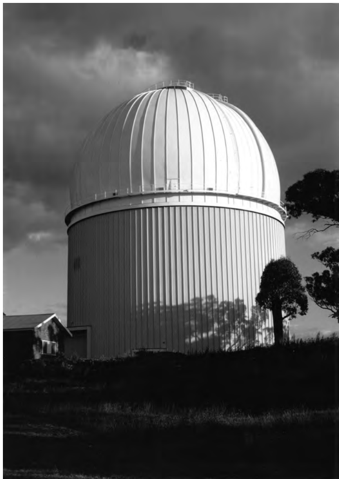
FIGURE 2 – Dome of the 3.9-m Anglo Australian Telescope near Coonabarabran N.S.W. The structure was designed to place the telescope high above thermal perturbations from the ground, but unfortunately with offices and laboratories and their heat sources in the intervening space. Peter Gillingham installed powerful fans to help equalize the outside air temperature with that around the telescope.
