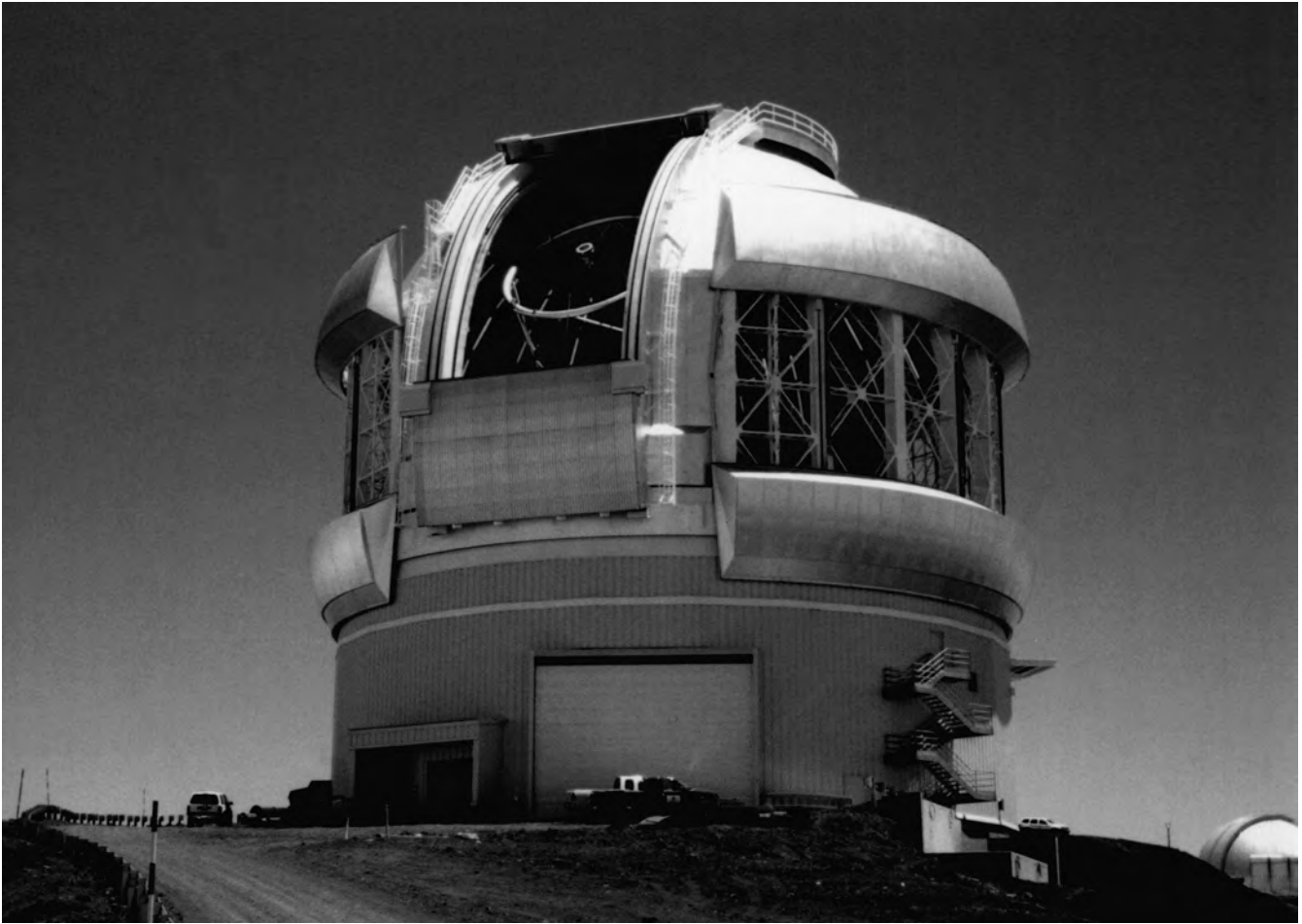
FIGURE 4 – The enclosure for the 8-m Gemini North Telescope showing the side panels open to enhance air circulation and hence minimize temperature gradients, which harm the seeing.
