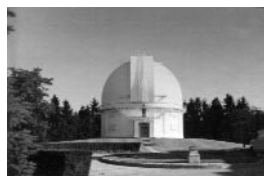
The dome for the 1.88-m telescope at the University of Toronto's David Dunlap Observatory.
