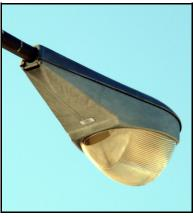
Fixtures like the cobrahead (top), and conehead (below) **waste up to 1/3 of their energy** into the night sky. Even semi-cut-off's, with a shallow-dish glass lens (diagram), produce light pollution and waste up to 5% of the energy produced. **Only full cutoff's prevent energy and light waste.**
